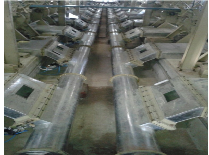
Intermittent Lint Suction System from Individual Double Roller Gin Machine
