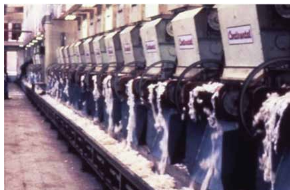
Figure 12. View of a single roller ginning plant
