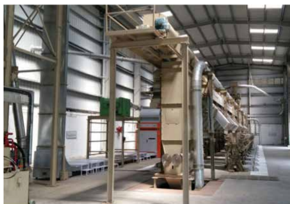
Figure 6. View of a double roller gin plant
