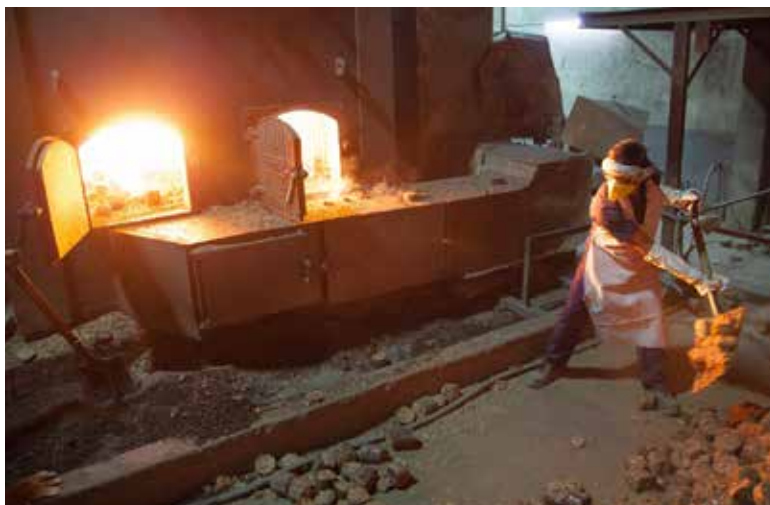
Figure 5. Briquette-fired boiler, Pix Transmission, MIDC Industrial Park, Hingna, Nagpur
