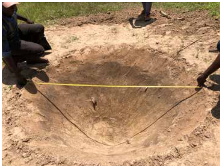
Figure-23. Conical pit of 2.0 meters diameter and 1.5 meters depth
