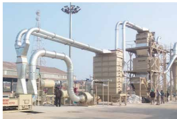
Figure 18. Cleaning & conveying setup for machine picked seed-cotton
