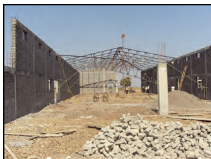
Figure 4: Particle Board Plant Under Construction at Washim, India
