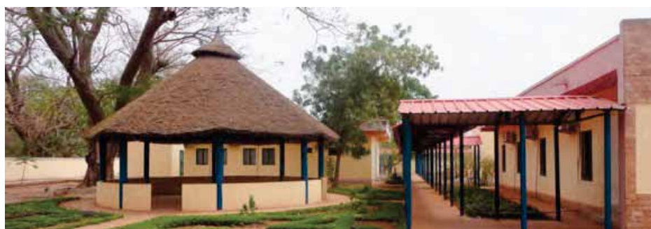
The C-4 Project Centre
